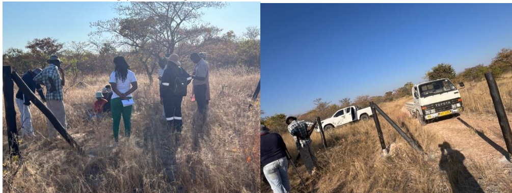
Figure 12 . The new fencing poles being erected at Nkankezi rangeland
