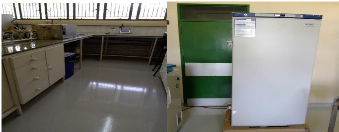
Plate 5.1: The Renovated Epoxy Floors and Scientific Laboratory Fridge
