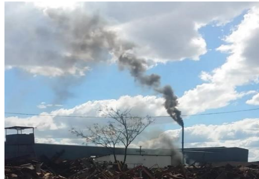
Plate 2.2: Black Stack and Fugitive Emissions From Panellink Furnace (21.04.2021).
